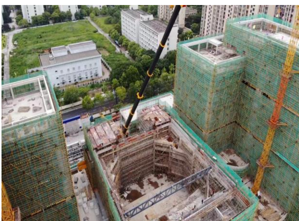
(钢结构桁架进场吊装)
