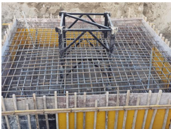
(塔吊基础施工)
