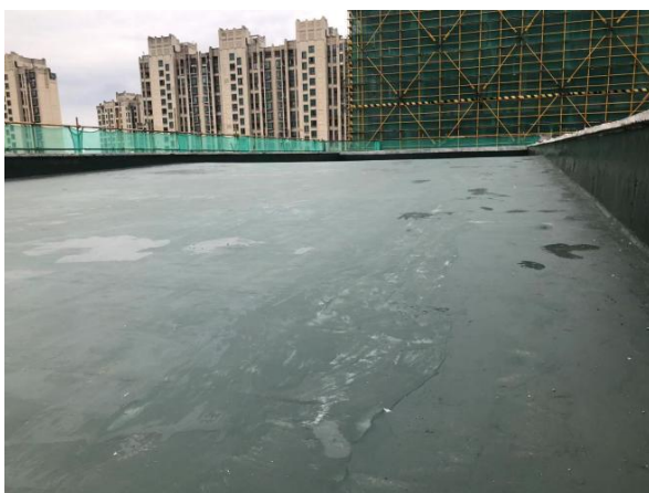
(B楼屋面防水涂料施工)
