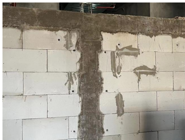
(圈梁构造柱浇筑)
