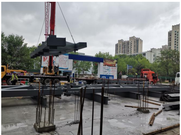
(钢结构桁架进场)
